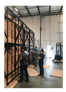
For the headquarters of a very large health care provider in New Jersey, Pierro and his PDS team addressed the challenges, with the integrator, of multiple LED arrays on one wall—they were all 11 feet high, but different widths, and they were all recessed into the wall.
